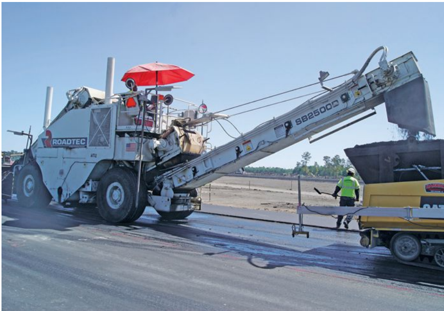
Barriere used a material transfer vehicle, skis and sensors to ensure the asphalt surface was smooth. With a 0.1-in. blanking band, they saw a profile index of 8.6 in. per mile.
