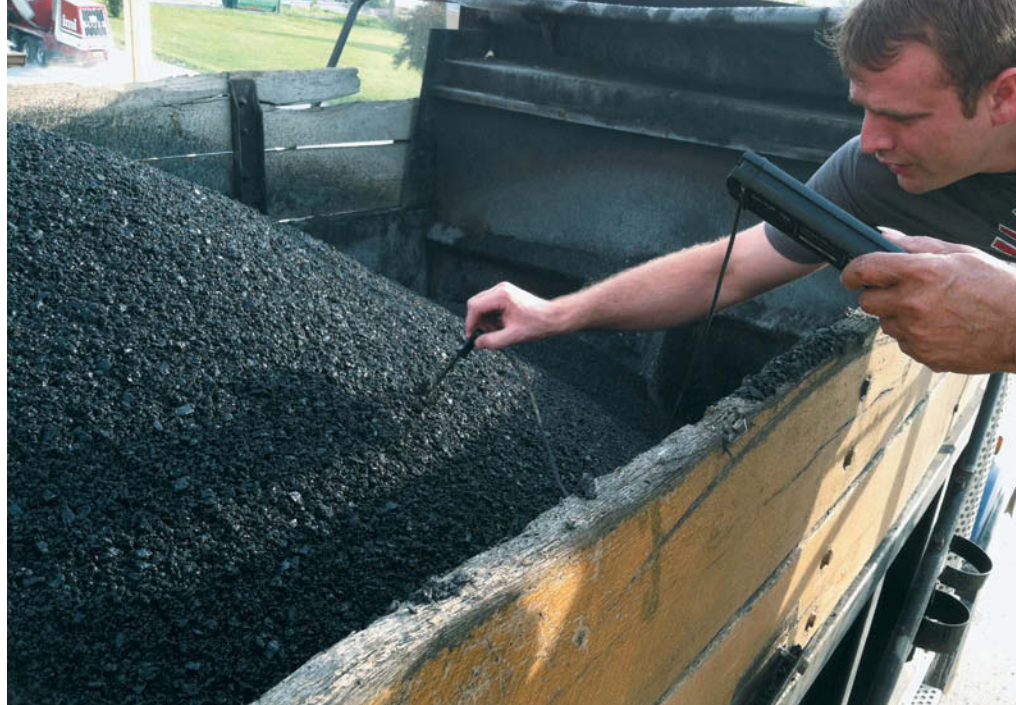
Quality control of every element of the modified surface mix was critical to the successful project. Photo credit: Advanced Material Services LLC
