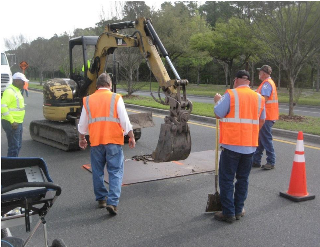
Removing steel plate over pavement depression
